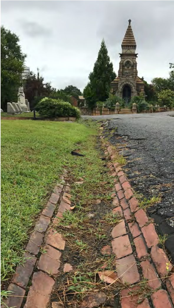
Some brick gutters have lost functionality over time due to sediment and vegetation
