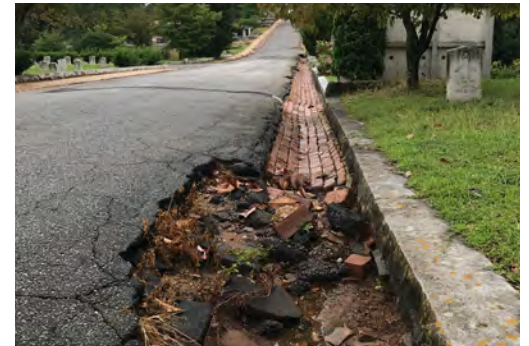
Top: Layers of asphalt rise above original brick gutters. Middle: Standing water leaves sediment at a broken inlet. Bottom: Failing asphalt road and gutter is no longer functional.
